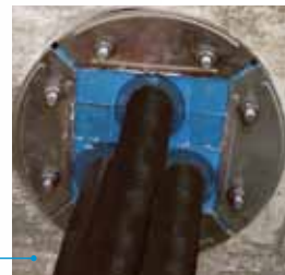
Transits for foundations.
