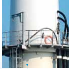
Transits for submarine cable in monopile.
