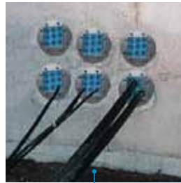
Transits into foundation.
