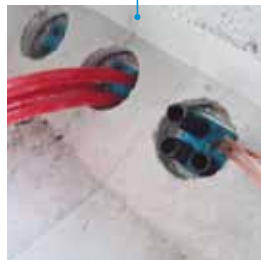
Transits for transformer shelters and transformer stations.
