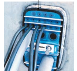
Frame with rounded corners (SRC) avoids cracks in the bulkheads around cable or pipe inlets.
