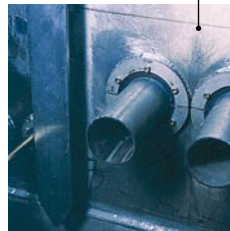
Roxtec RS seals for pipes in main engine room.
